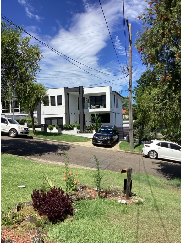
Figure 10 Modern development on Hilltop Avenue
